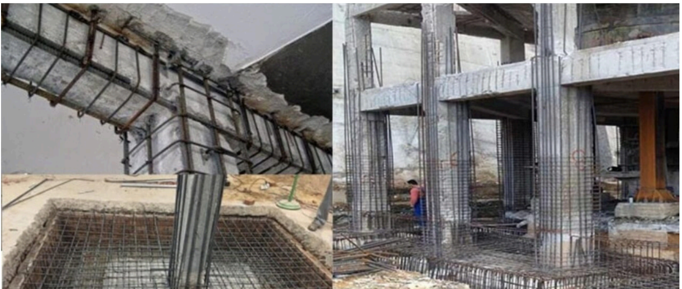
Retrofitting of RC Structures
